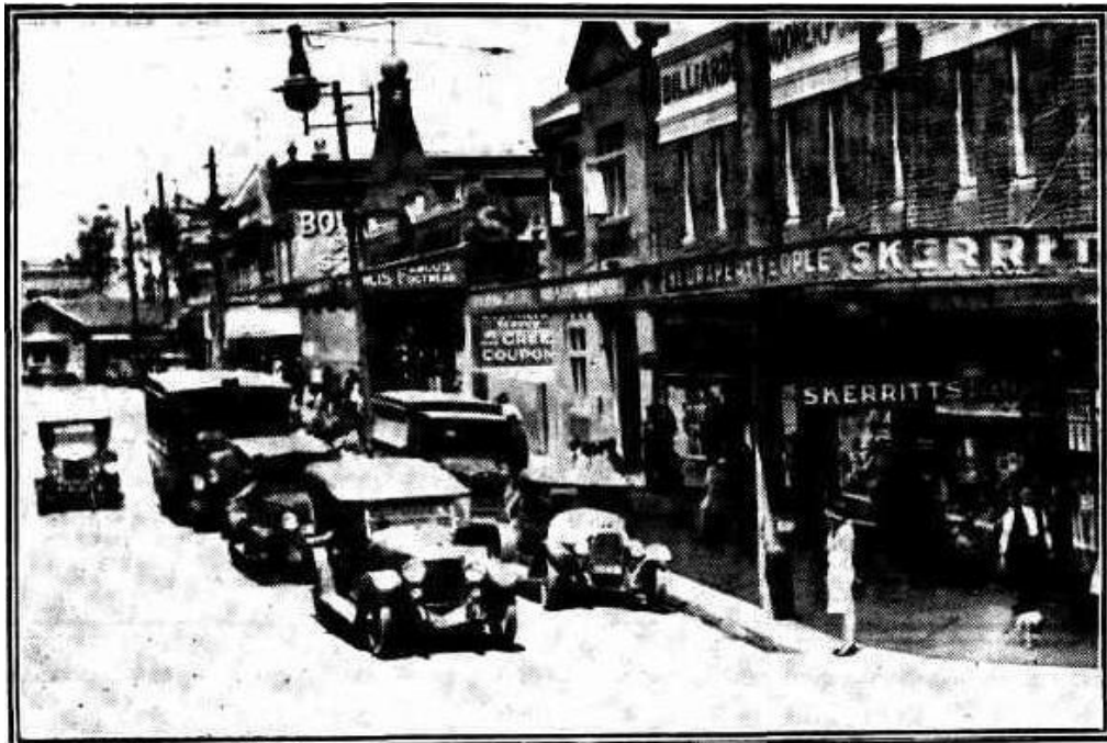
Figure 14 — Good Street, Granville looking south from Sydney (Parramatta) Road. 36-42 Good Street on right with Turret of Patten’s building clearly visible beyond and the enlarged Fire Station in between. (Source: Cumberland Argus and Fruitgrowers Advocate, 12 December 1929, p2)
